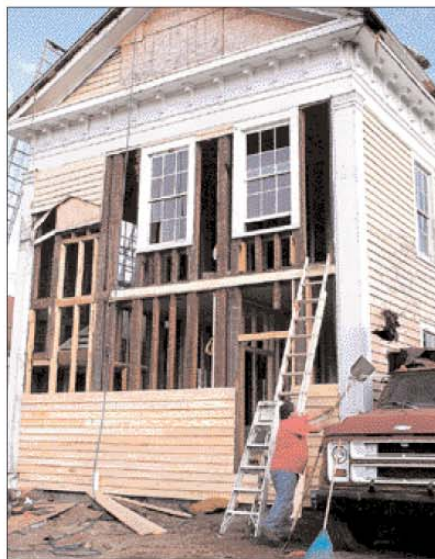
Antonio Rojas shovels roofing debris.
